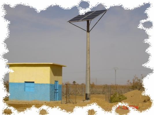
**Figure 08: Setting of the solar energy for the water pumping in rangeland (Ain Naga, Algeria)**
